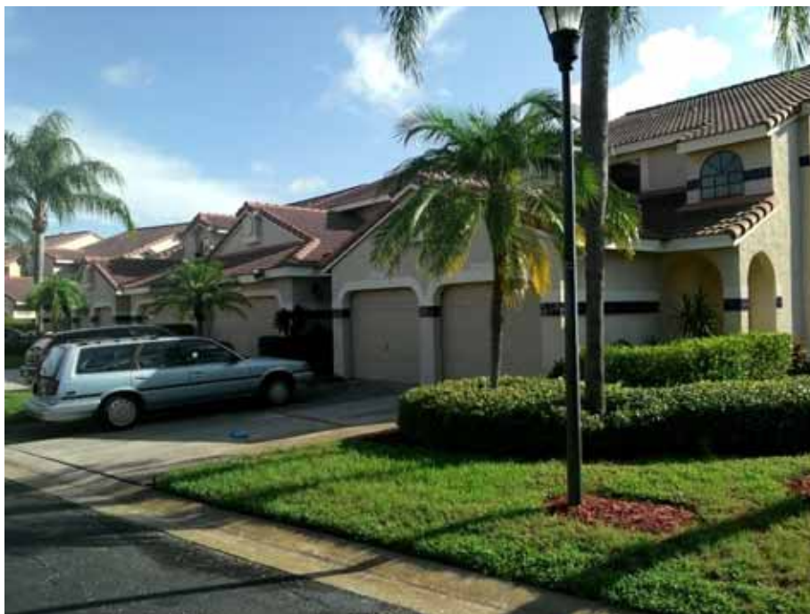
10413-10423 St. Tropez Pl (Condo Bldg, 6 Units)
