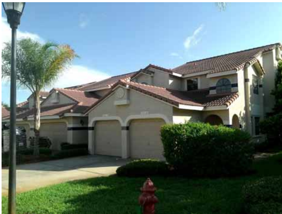
10425-10435 St. Tropez Pl (Condo Bldg, 6 Units)
