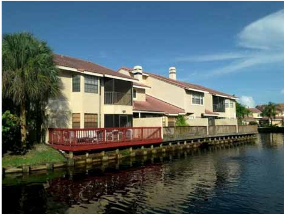
10425-10435 St. Tropez Pl (Condo Bldg, 6 Units)
