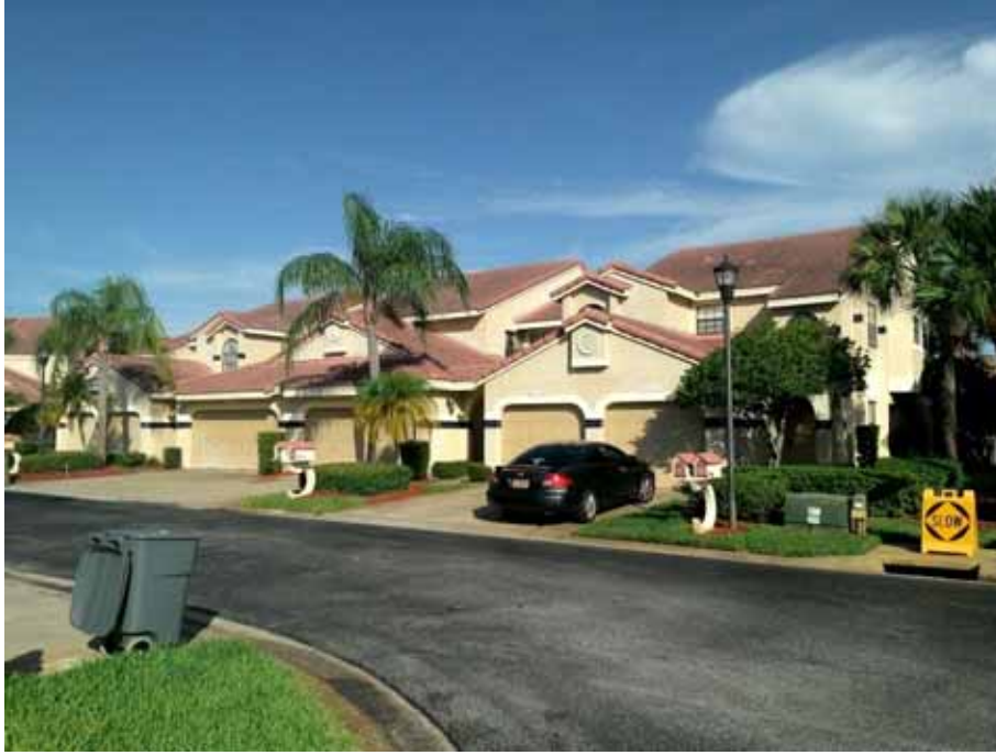
10472-10482 St. Tropez Pl (Condo Bldg, 6 Units)
