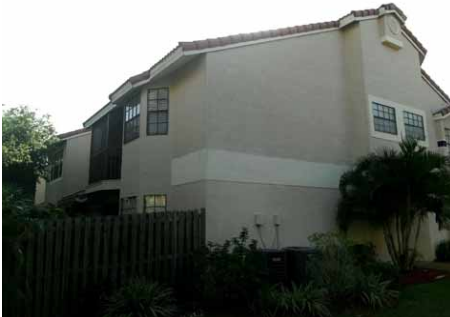
10472-10482 St. Tropez Pl (Condo Bldg, 6 Units)
