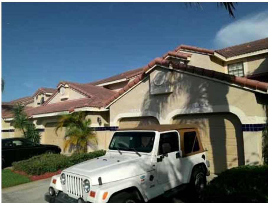
10484-10494 St. Tropez Pl (Condo Bldg, 6 Units)
