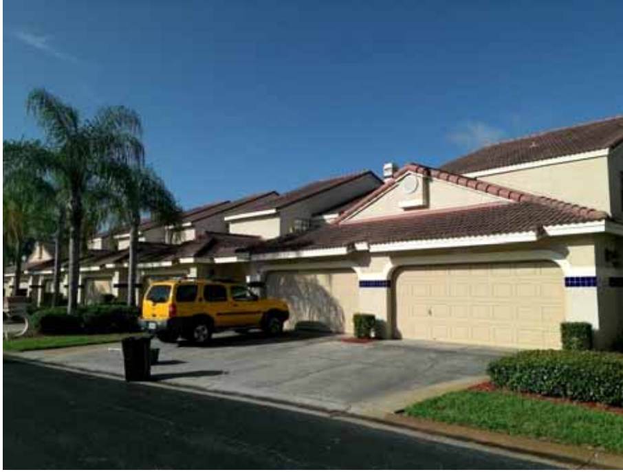
10412-10424 St. Tropez Pl (Condo Bldg, 7 Units)
