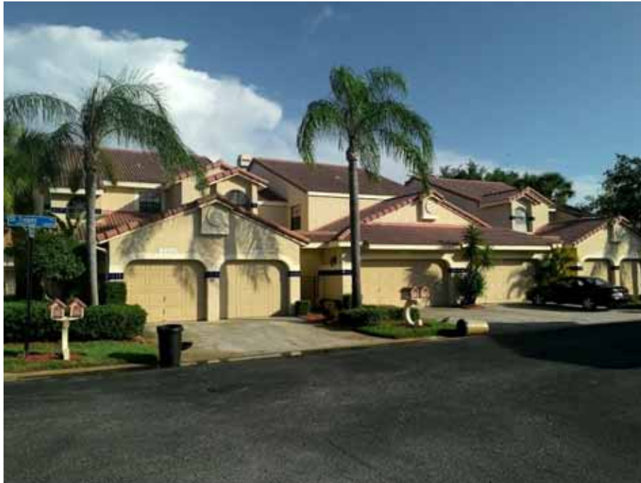
10484-10494 St. Tropez Pl (Condo Bldg, 6 Units)
