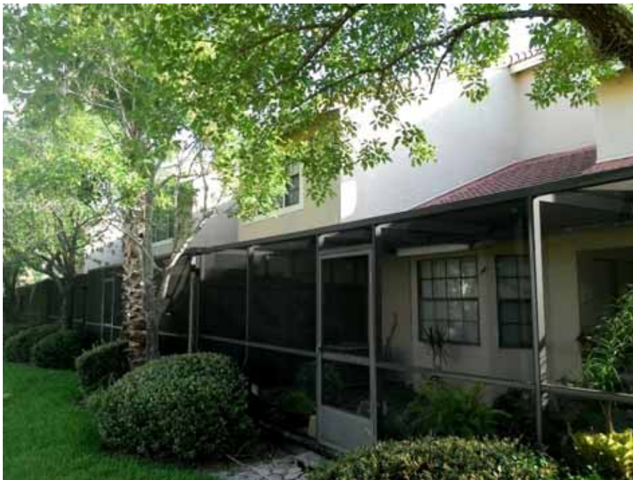
10412-10424 St. Tropez Pl (Condo Bldg, 7 Units)
