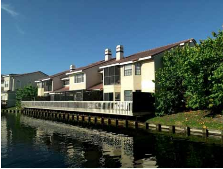
10413-10423 St. Tropez Pl (Condo Bldg, 6 Units)
